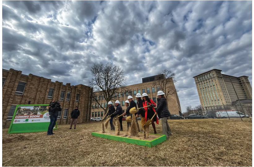
Kintsugi Village kicked off construction Wednesday with a groundbreaking for a community hub in Corktown that will house an early childhood education center, an artist incubator and other services. David Guralnick, The Detroit News
